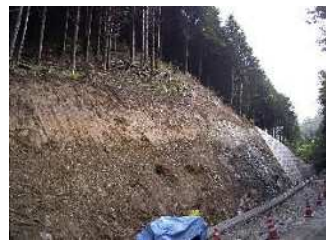
①法面清掃
